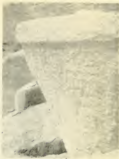
FIG. 9.—ROUGH CHISEL-DRESSING ON UNFINISHED SARCOPHAGI KNOWN AS "EL-HAMMÂMMÂT" NEAR ASWAN. (Page 31.)
