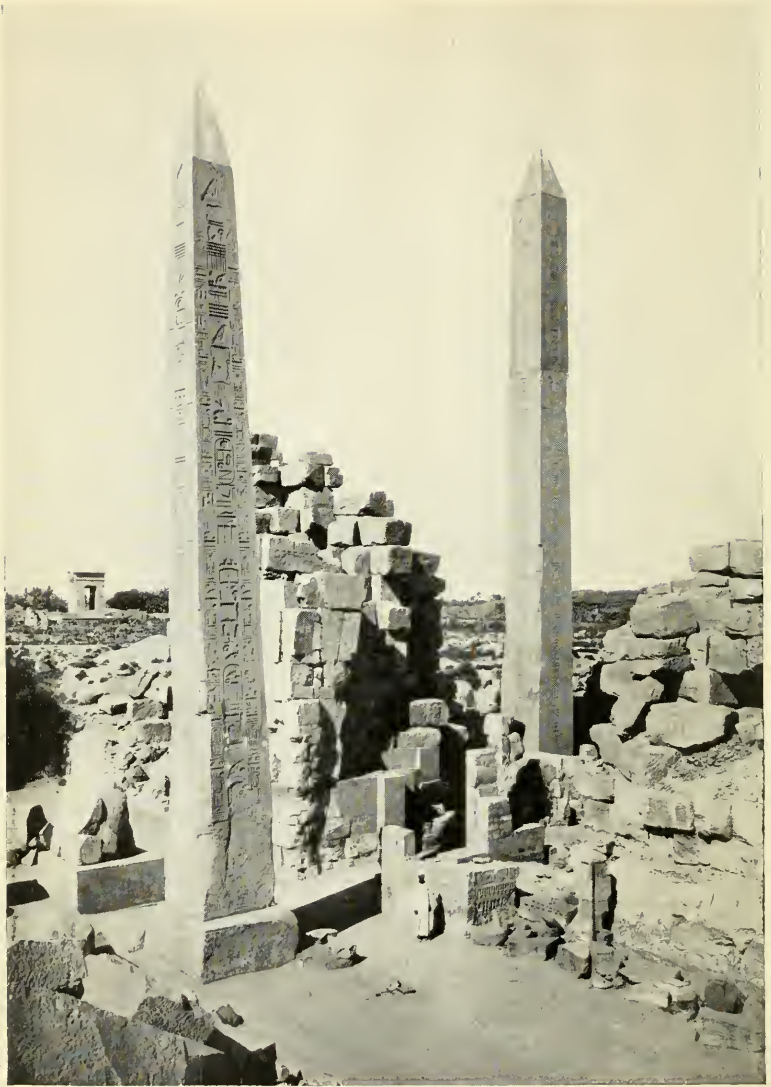
FIG. 1.—OBELISKS OF TUTHMÔSIS I (left) AND HATSHEPSOWET (right) AT KARNAK. (The nearer obelisk leans to the left owing to soil-subsidence.)
