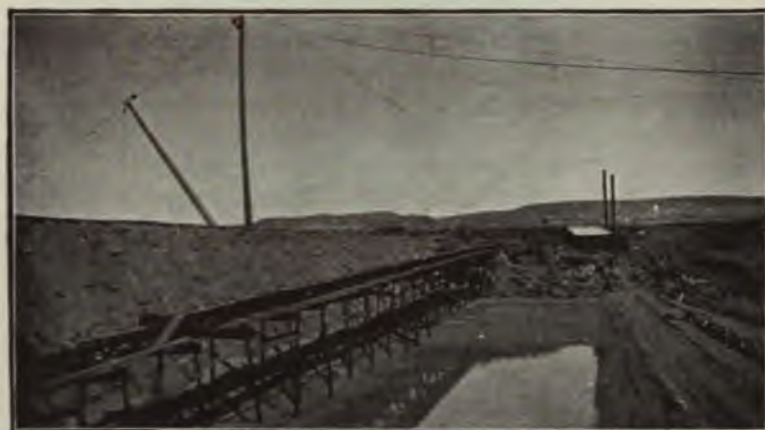
FIG. 59.—ZUÑI DAM, N. M., ILLUSTRATING METHOD OF DELIVERY OF SLUICED MATERIALS BY "V" FLUME, AGAINST FACE OF ROCK-FILL.
