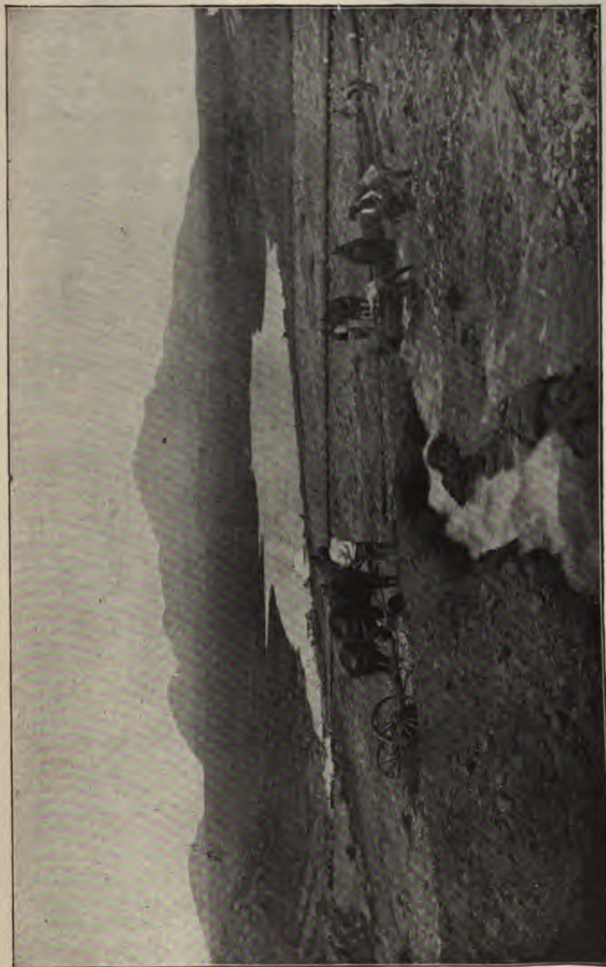
FIG. 71.—LA MESA (CAL.) DAM IN COURSE OF CONSTRUCTION BY THE HYDRAULIC PROCESS. Showing method of loosening earth to get it in suspension before taking it into carrying conduit. The conduit was built in 24-foot sections, which could be and were frequently taken apart and moved as conditions required.
