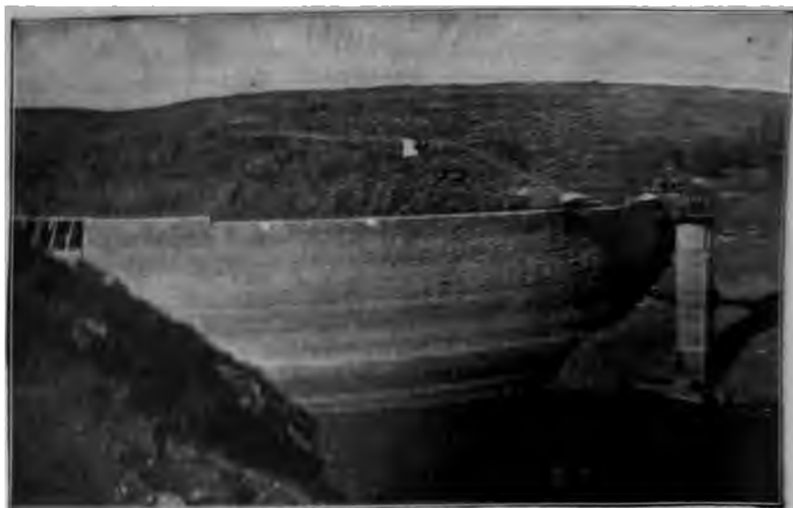
FIG. 152. FACE OF SWEETWATER DAM IN 1899. AFTER TWO YEARS OF DECAY.
