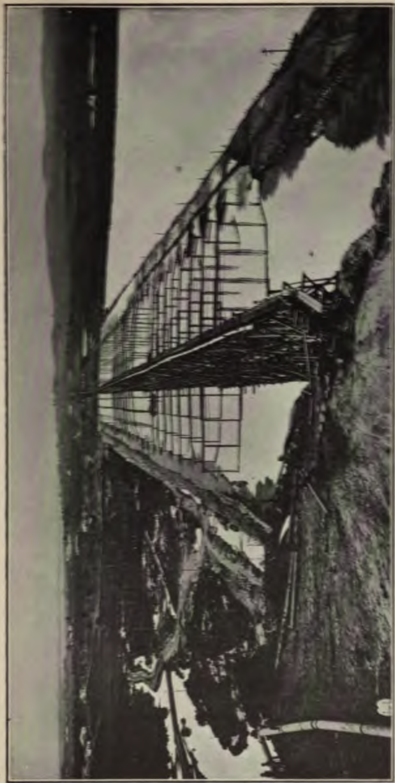
FIG. 109.—SANTO AMARO DAM, SÃO PAULO, BRAZIL. (1 MILE LONG.) SHOWING METHOD OF DELIVERY OF SLICED MATERIAL THROUGH FLUMES AND LATERALS.
