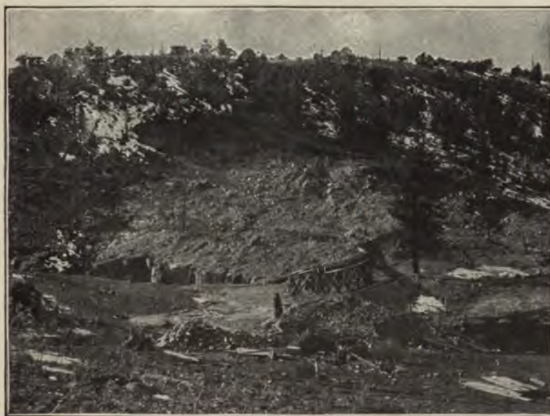
FIG. 105.—TERRACE DAM. DEPOSIT OF HYDRAULIC FILLING ON THE UPPER TOE SLOPE.
