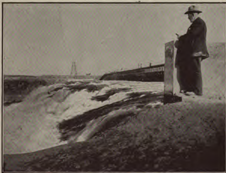
FIG. 48.—MILNER DAM, SNAKE RIVER, IDAHO. SHOWING WASTE-WAY GATES AND DISCHARGE OF RIVER OVER "IRRIGATION FALLS."
