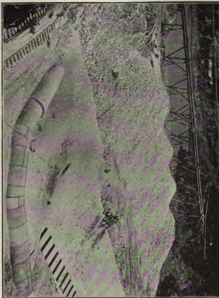
FIG. 126.—LOWER TOE OF NECACAXA DAM, MEXICO, SHOWING CHARACTER OF HYDRAULIC-FILL MATERIAL. PIPE IN FOREGROUND IS 10 FEET IN DIAMETER, USED ONLY FOR FLOOD DISCHARGE DURING CONSTRUCTION.
