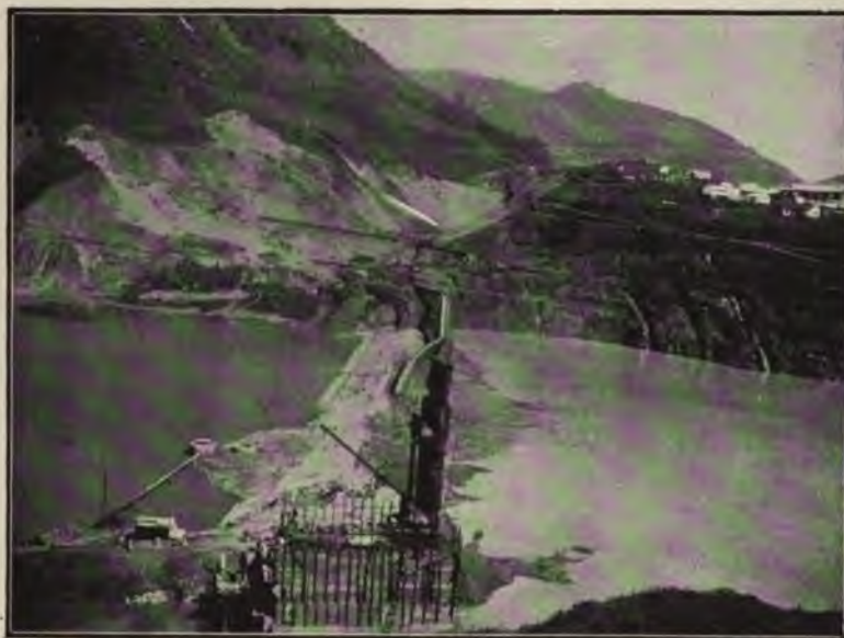
FIG. 124.—NECAXA DAM, UP-STREAM SLOPE, LOOKING TOWARD SLUICING PIT AND SPILLWAY GAP.
