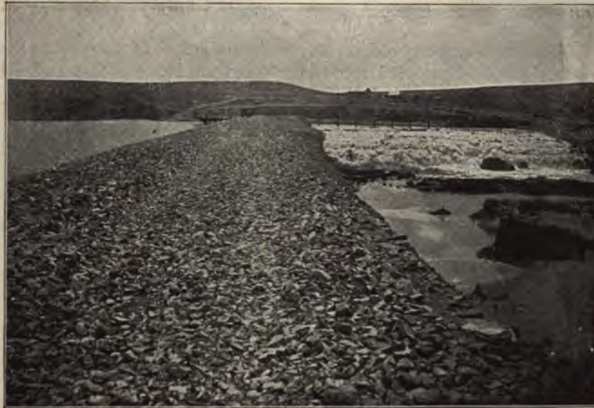
FIG. 34.—LAKE AVALON DAM, PECOS RIVER, NEW MEXICO. SHOWING THE CREST OF COMPLETED DAM AND SPILLWAY DISCHARGING.
