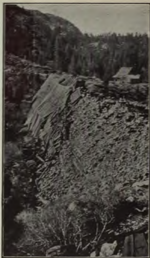
FIG. 346.—UP-STREAM FACE OF ONE OF THE TWO REMAINING ROCK-FILL STRUCTURES WHICH, WITH THE THIRD STRUCTURE DESTROYED IN 1883, ORIGINALLY FORMED THE ENGLISH LAKE DAM.
