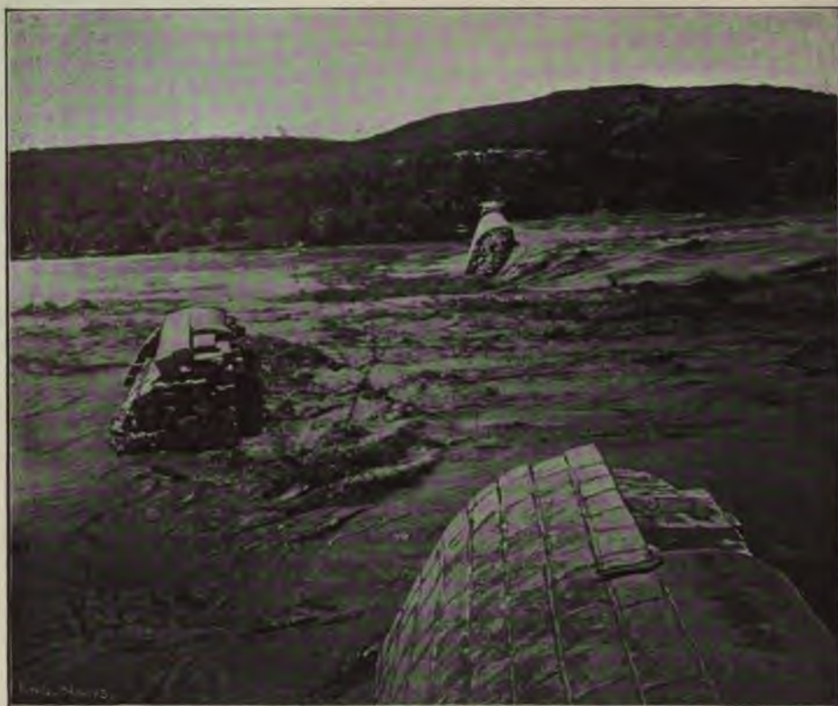
FIG. 230.—AUSTIN DAM, TEXAS. VIEW TAKEN DURING FLOOD, A FEW MINUTES AFTER THE BREAK
