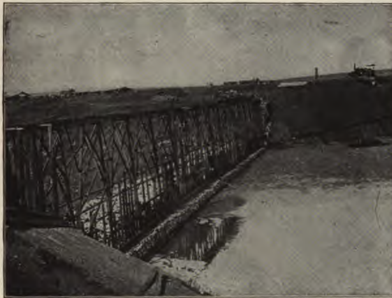
FIG. 95.—WAIALUA DAM, SHOWING HYDRAULIC-FILL BEING SLUICED IN AGAINST THE ROCK-FILL.
