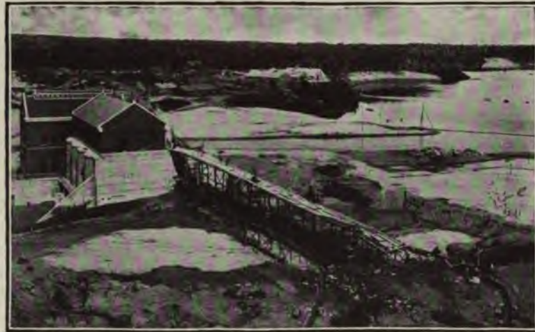
FIG. 137.—CROTON HYDRAULIC-FILL DAM, MICHIGAN, DURING CONSTRUCTION.
