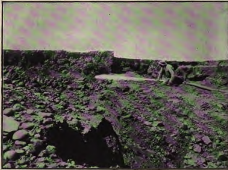
FIG. 134.—YORBA DAM, CALIFORNIA. HYDRAULICKING AN EARTH BANK WITH WATER PUMPED THROUGH 1-INCH NOZZLE UNDER 25 POUNDS PRESSURE.
