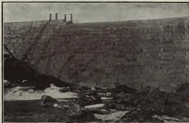
FIG. 63.—ALFRED DAM, ME. DRY ROCK MASONRY WITH CONCRETE FACING AND CREST.
