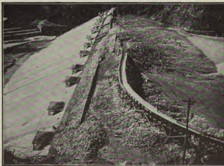
FIG. 121.—DOWN-STREAM SLOPE OF NECAXA DAM, SHOWING MASONRY PAVEMENT ON FACE AND CHARACTER OF SLICED MATERIAL.
