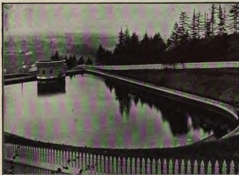
FIG. 211.—RESERVOIR NO. 1, PORTLAND, ORE., WATERWORKS. CONCRETE DAM WITH EARTH BACKING.
