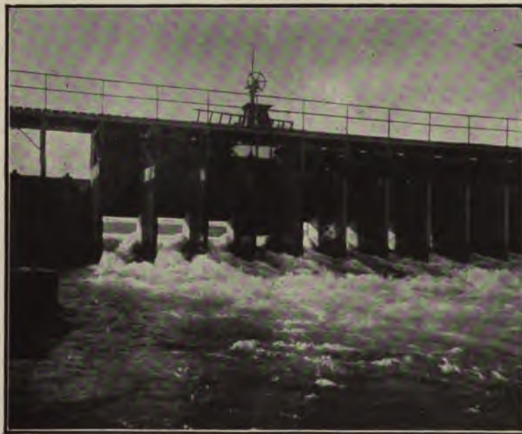
FIG. 52.—MILNER DAM, IDAHO. SHOWING A PART OF THE BATTERY OF 99 WASTE-GATES.
