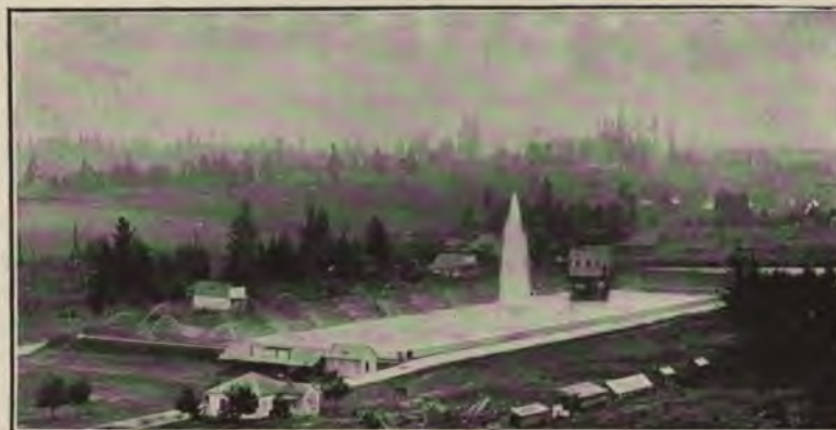
FIG. 216.—RESERVOIR NO. 2, PORTLAND, OREGON, WATERWORKS, SHOWING AERATION FOUNTAINS.
