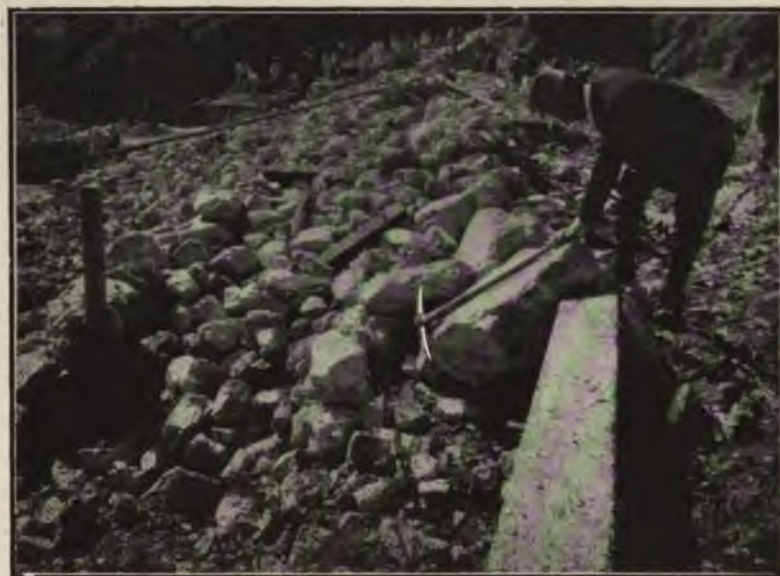
FIG. 119.—ILLUSTRATING THE SIZE OF STONE DELIVERED BY FLUME TO THE NECAXA DAM. THE LARGEST ONE MEASURED CONTAINED 18 CUBIC FEET.
