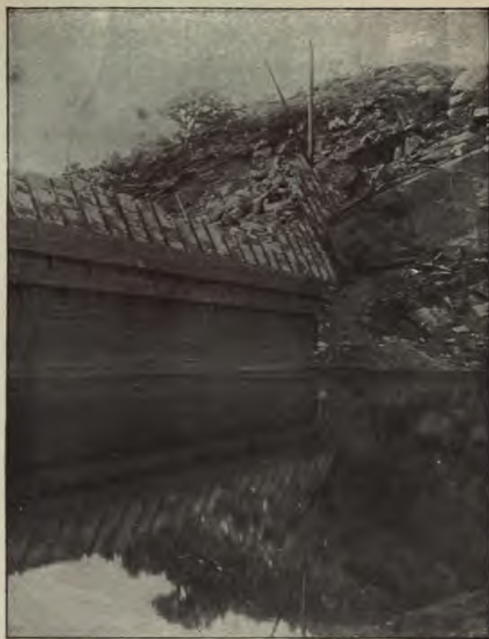
FIG 9.—CONSTRUCTION OF FACING OF ESCONDIDO DAM.
