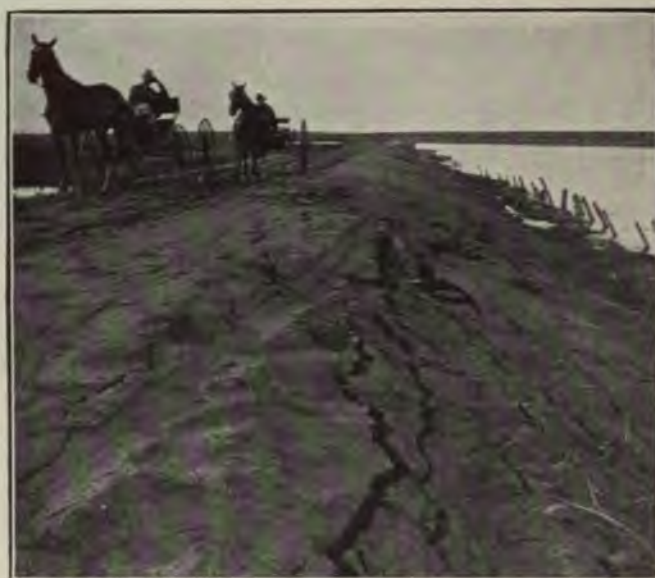
FIG. 333.—DOUGLAS LAKE DAM, COLORADO, SHOWING DANGEROUS SETTLEMENT CRACKS, DUE TO IMPROPER METHOD OF CONSTRUCTION.
