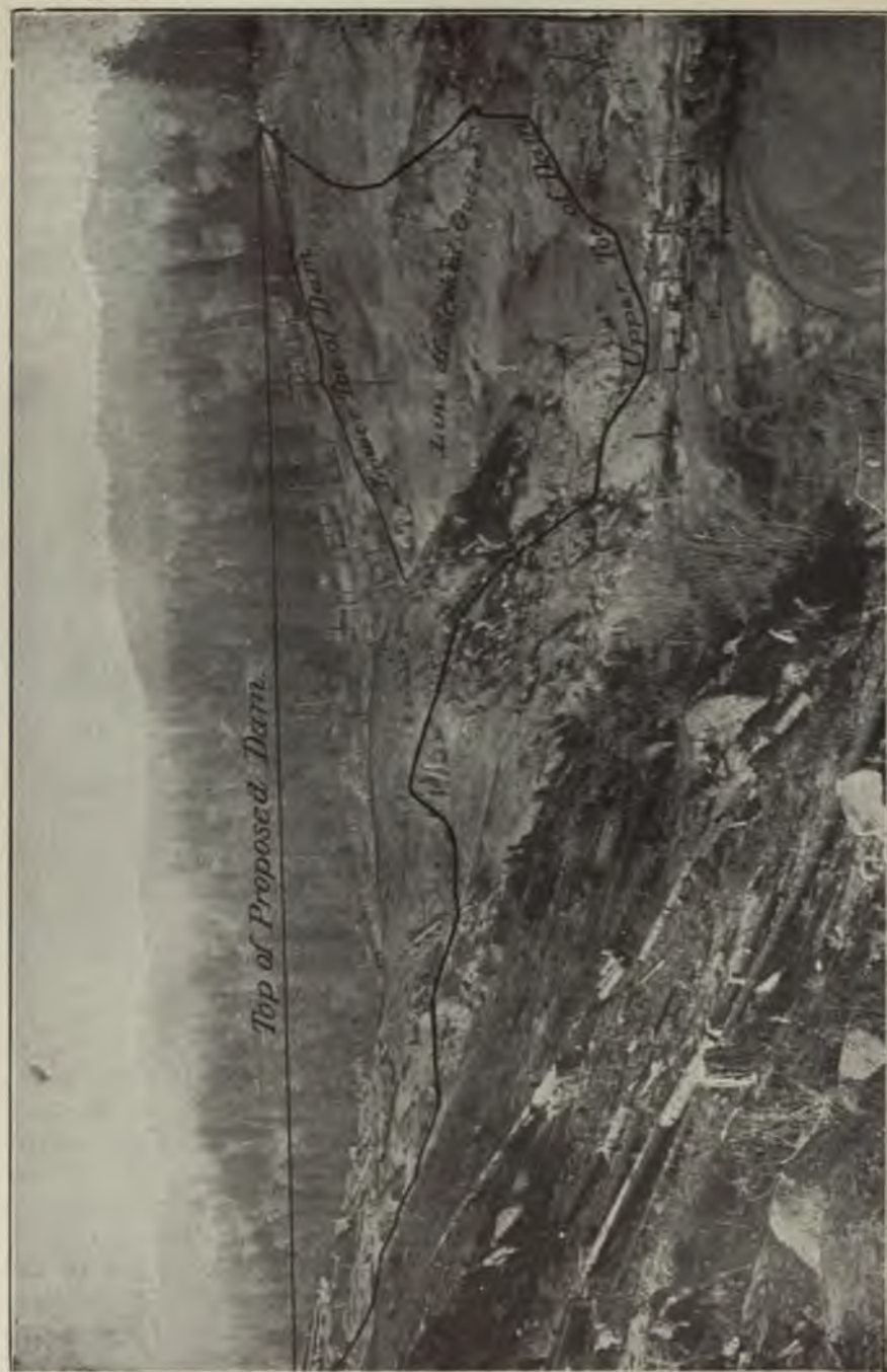
FIG. 77.—VIEW OF CRANE VALLEY DAM-SITE, SHOWING OUTLINES OF HYDRAULIC-FILL DAM.
