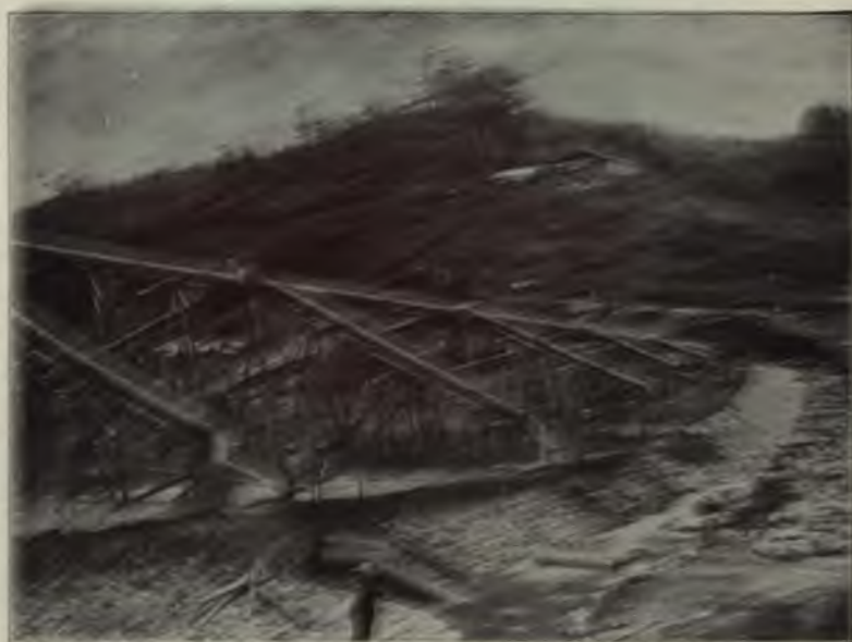
FIG. 130.—LIQUID EARTH BEING DEPOSITED THROUGH PIPES ON OUTER SLOPE OF DAM NO. 1, TENANGO RIVER.
