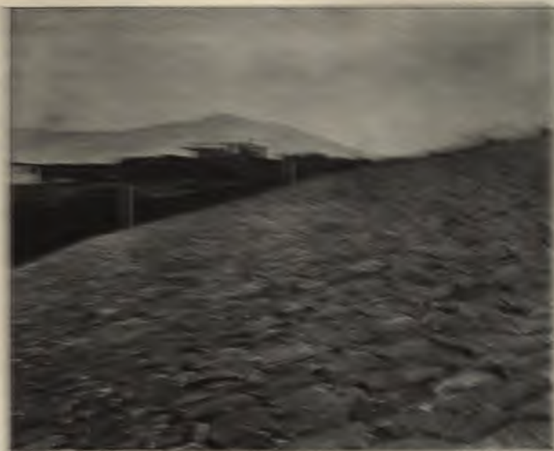
FIG. 98.—REPAIR ON FACE OF HYDRAULIC-FILL, WAIALUA DAM.
