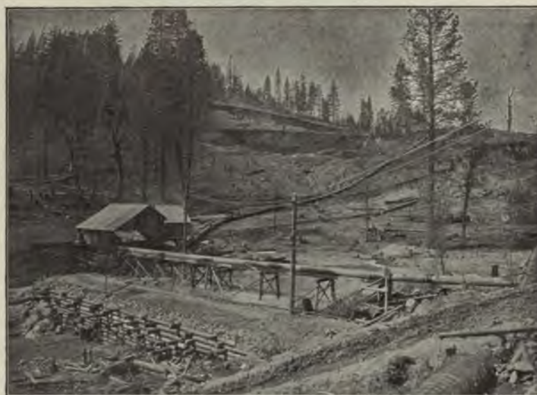
FIG. 91.—LAKE FRANCES DAM CONSTRUCTION. PUMPING STATION, SHOWING SUCTION PIPE CONNECTED TO TANDEM CENTRIFUGAL PUMP. CRIB DAM IN FOREGROUND BUILT TO STORE WATER FOR EARLIER OPERATIONS.
