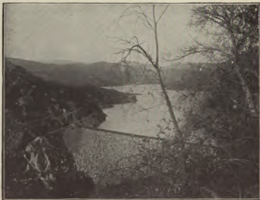
FIG. 10.—ESCONDIDO (CAL.) ROCK-FILL DAM. WOODEN LINING.
