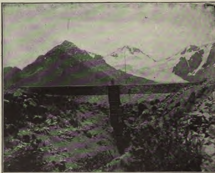
FIG. 277.—CARPA DAM, PERU, SHOWING TYPICAL OUTLET CUT, FILLED WITH STEEL BULKHEAD, GLACIER IN BACKGROUND.
