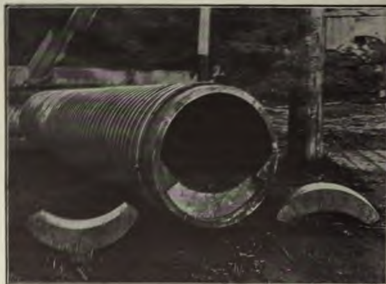
FIG. 350.—THE HOPKINS WOOD PIPE, FOR CARRYING GRITTY MATERIAL, THE WEAR BEING UPON THE END GRAIN OF THE WOOD.
