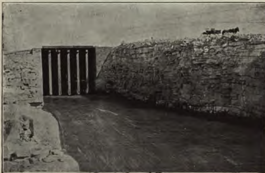
FIG. 35.—CANAL HEADGATES, LAKE AVALON DAM.
