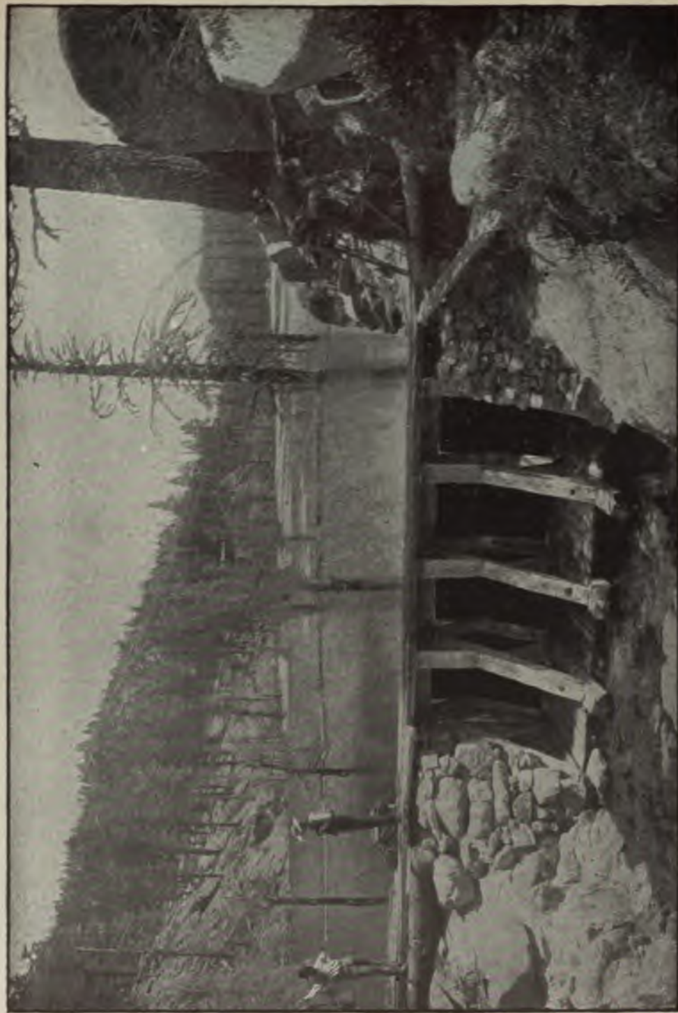
FIG. 175.—SPILLWAY OF BEAR VALLEY DAM, WITH FLASHBOARD GATES.
