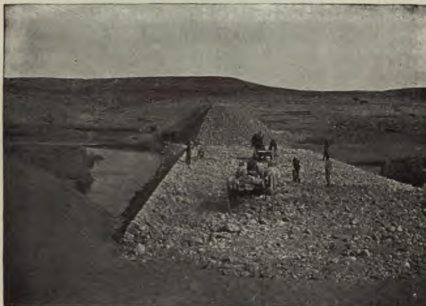
FIG. 33.—LAKE AVALON DAM. ROCK-FILL IN PROCESS OF CONSTRUCTION.
