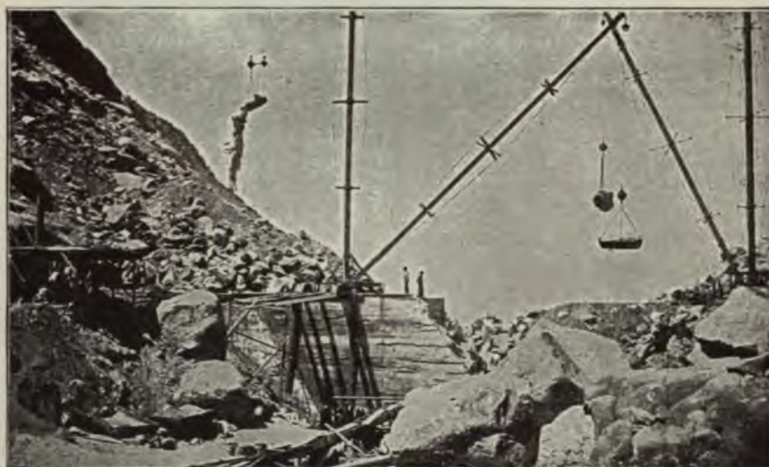
FIG. 23.—MORENA ROCK-FILL DAM, SHOWING A PORTION OF TOE-WALL UNDER CONSTRUCTION.
