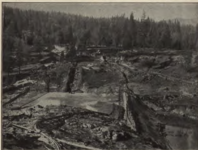
FIG. 82.—BORROW-PITS FROM WHICH MATERIAL WAS SLUCED TO THE CRANE VALLEY DAM IN BACKGROUND.
