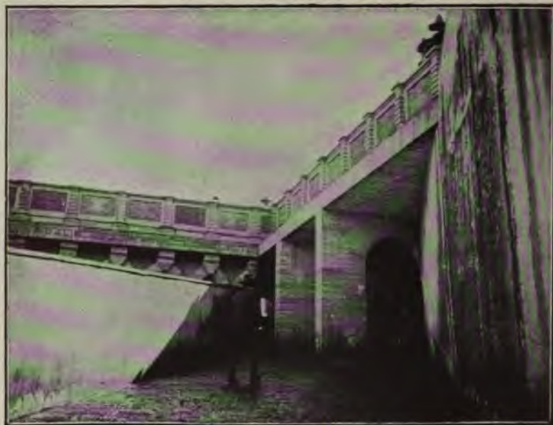
FIG. 365.—THE SPILLWAY CHANNEL OF THE ESPERANZA DAM, AT ITS UPPER END, SHOWING OBSTRUCTIONS TO FREE DISCHARGE BY PIERS SUPPORTING ROADWAY.
