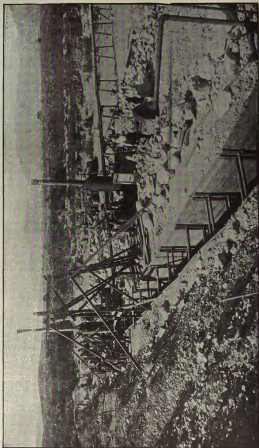
FIG. 196.—EXCAVATION OF TRENCH FOR PACOIMA SUBTERRANEAN DAM.
