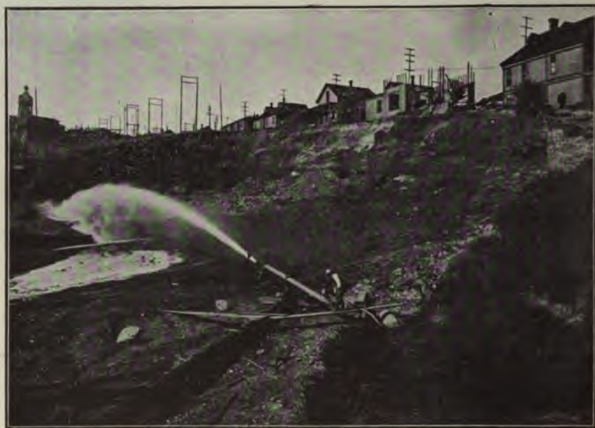
FIG. 352.—THE REGRADING OF JACKSON STREET, SEATTLE, LOOKING NORTH ON MAYNARD STREET. THE HOUSES ARE REMOVED JUST BEFORE THEY ARE UNDERMINED.
