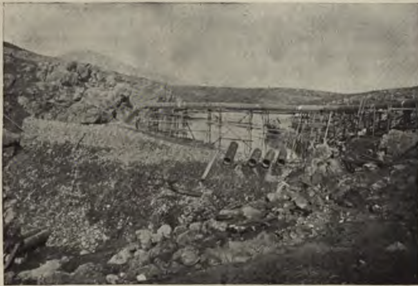
FIG. 76.—LA MESA HYDRAULIC-FILL DAM, SHOWING PIPE DISCHARGING MATERIAL ON THE DAM.
