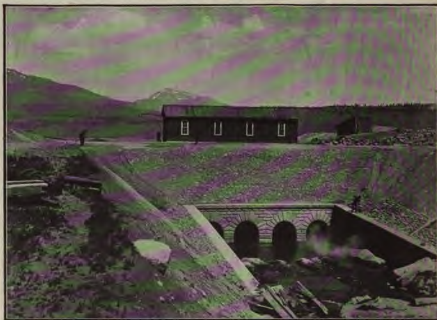
FIG. 331.—TWIN LAKES, COLORADO, MASONRY DAM OVER OUTLET, WITH EARTH BACKING, GATE-HOUSE, AND OUTLET CULVERTS.
