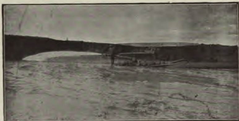
FIG. 60.—ZUÑI DAM, NEW MEXICO, SHOWING HYDRAULIC MONITOR IN ACTION.
