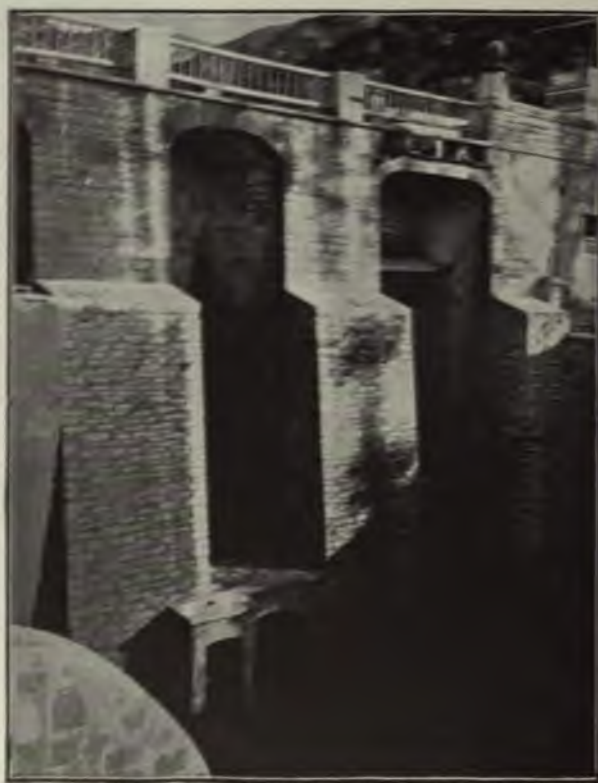
FIG. 370.—A DETAIL OF THE DOWN-STREAM FACE OF THE LOWER OLLA DAM, GUANAJUATO. These openings are closed by a form of movable flash-board.
