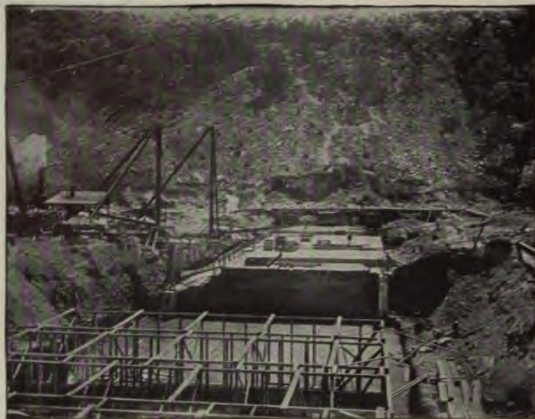
FIG. 322. —WHEEL PIT AND CUT-OFF WALLS, JUNIATA DAM.
