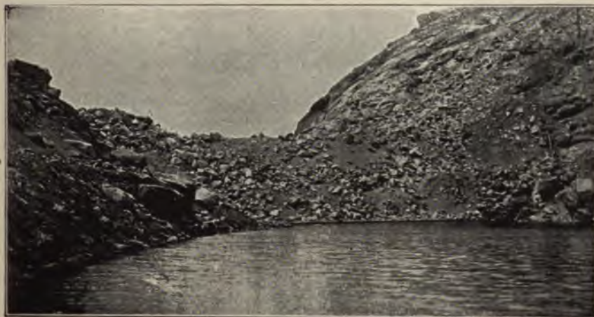
FIG. 22.—MORENA ROCK FILL DAM IN PROCESS OF CONSTRUCTION. SHOWING TOP OF TOE-WALL ABOVE THE WATER-LINE.
