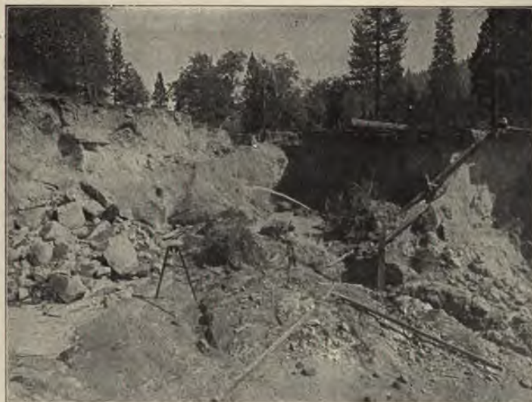
FIG. 81.—CRANE VALLEY HYDRAULIC-FILL DAM. SHOWING METHOD OF LOOSENING THE MATERIALS SLUICED INTO THE DAM.
