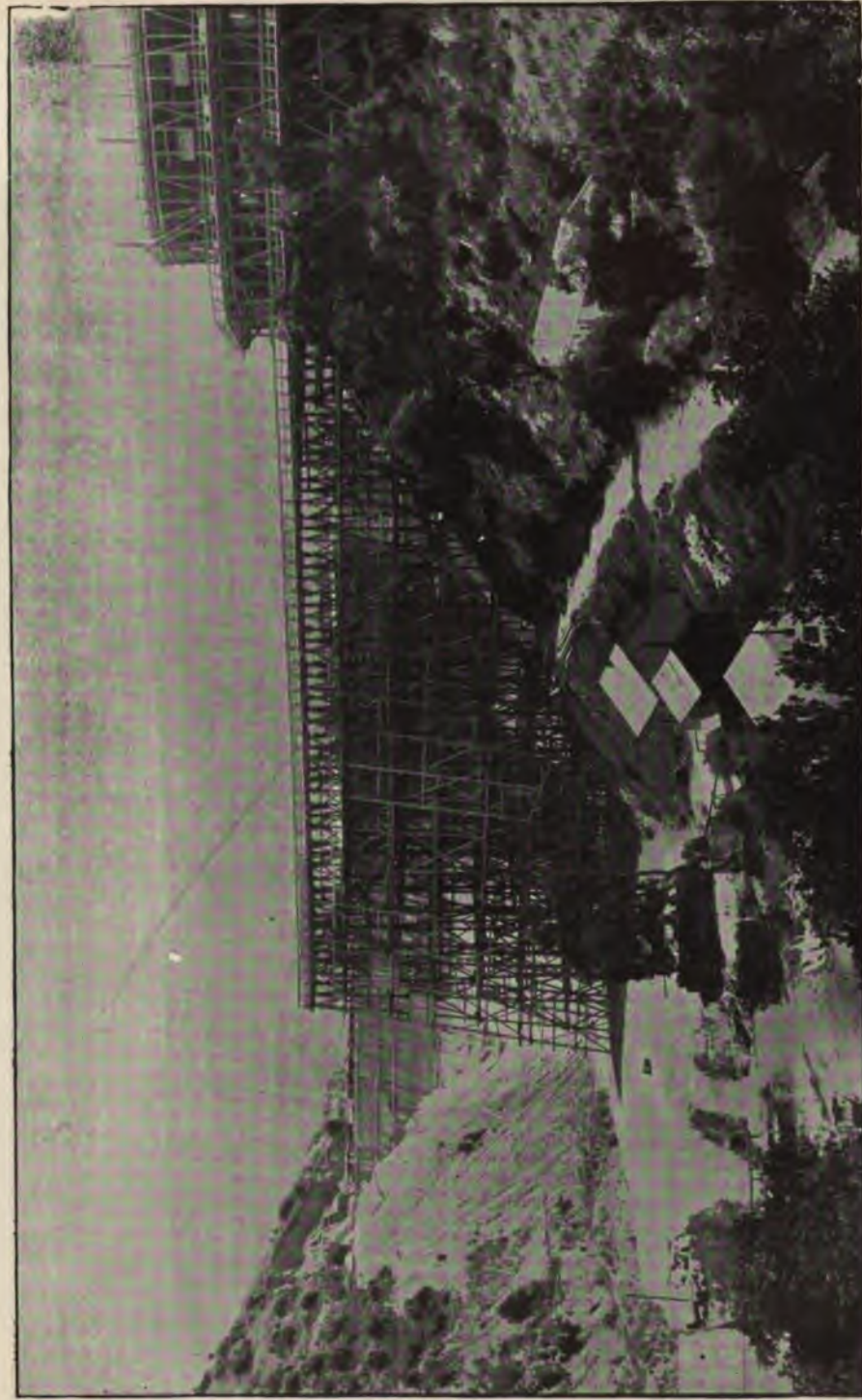
FIG. 190.—PLANT FOR MIXING AND HANDLING CONCRETE AT SAN MATEO DAM.
