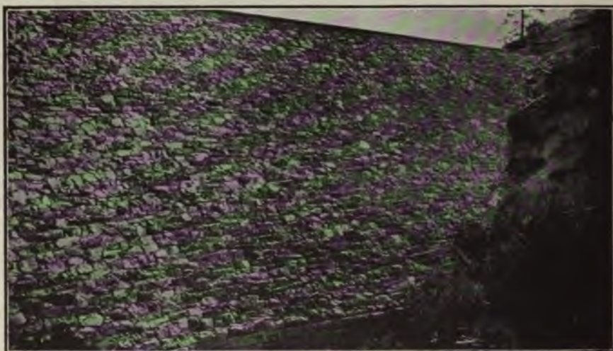
FIG. 338.—DOWN-STREAM FACE OF BOWMAN LAKE DAM, CALIFORNIA, ILLUSTRATING THE QUALITY OF THE DRY MASONRY.
