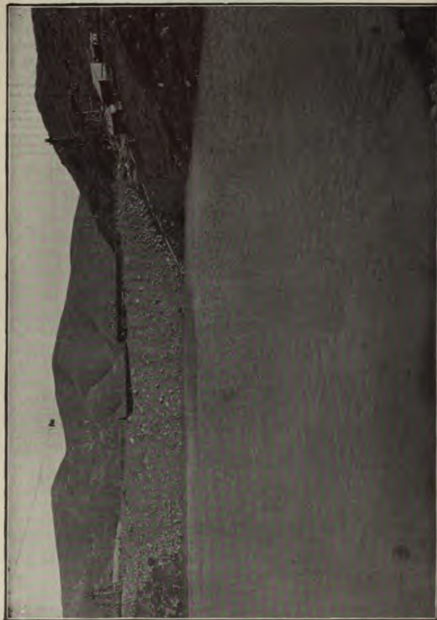
FIG. 12.—OTAY (CAL.) ROCK-FILL DAM—STEEL CORE.
