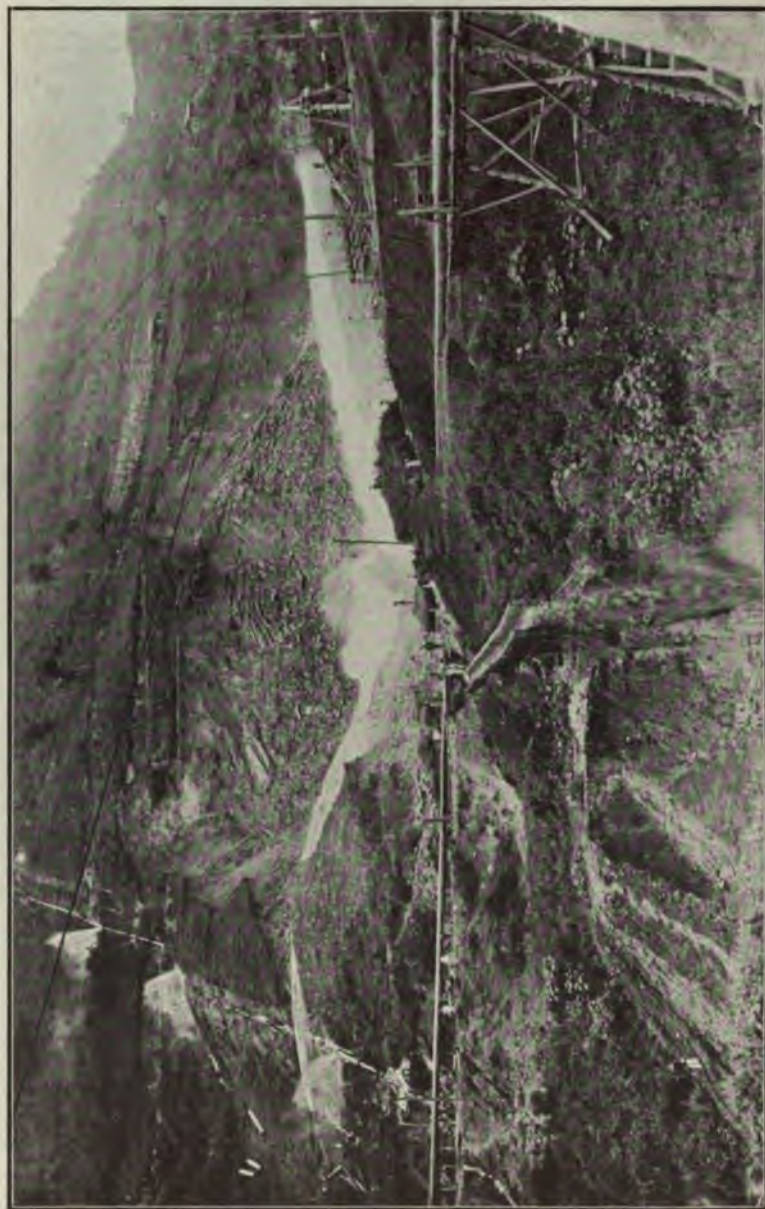
FIG. 127.—HYDRAULIC SLUICING AT NECAXA, JUNE, 1907. SHOWING TILTED LIMESTONE LEDGES IN PIT NO. 1, OVERLAID BY CLAY AND LOOSE ROCK.
