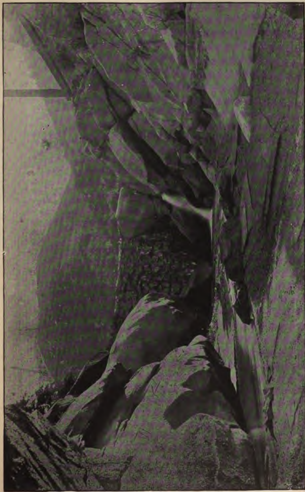
FIG. 20.—THE BARRETT DAM-SITE, SHOWING THE BEGINNING OF MASONRY FOUNDATIONS. The material on left bank above the rock here shown is disintegrated granite to such depth as to require change of plans from original design.
