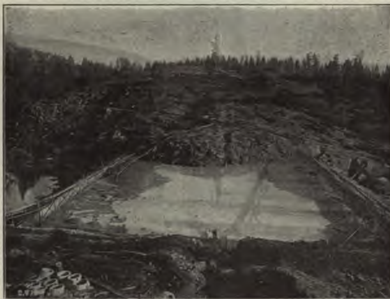
FIG. 80.—CRANE VALLEY DAM SHOWING DISCHARGE OF SLUCED EARTH AT END OF CONVEYING FLUME.
