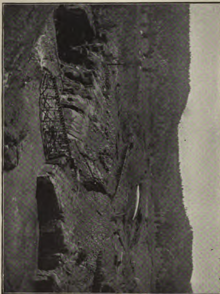
FIG. 107.—VIEW OF LOWER TOE FILLING, TERRACE DAM, COLORADO, SHOWING HYDRAULIC SLUICING IN BACKGROUND.
