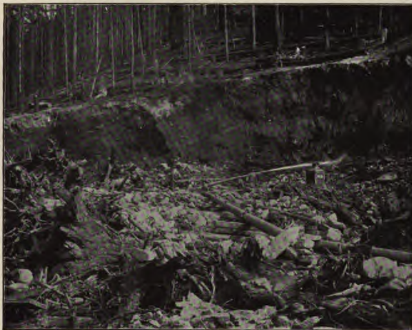
FIG. 145.—NORTHERN PACIFIC RAILWAY, HYDRAULIC-FILL CONSTRUCTION. VIEW IN PIT SHOWING HYDRAULIC GIANT IN ACTION.
