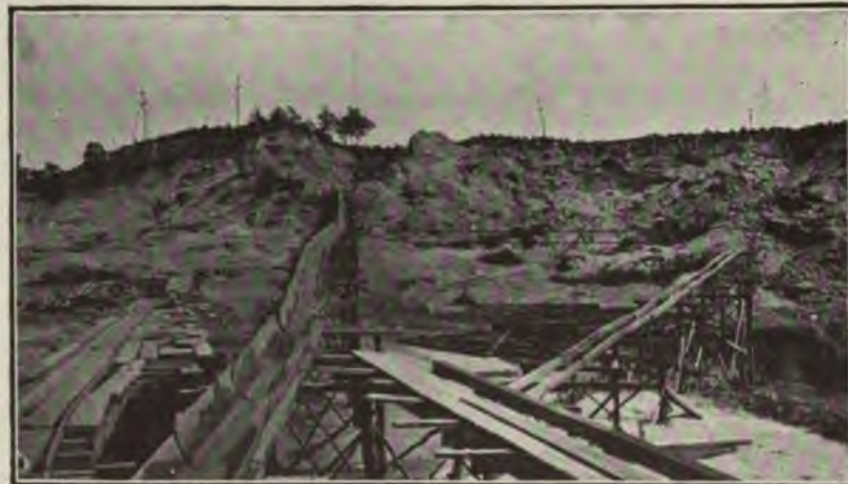
FIG. 138.—CROTON DAM, MICHIGAN, ILLUSTRATING FLUMES AND TRESTLE SUPPORTS USED IN HYDRAULIC SLUICING.
