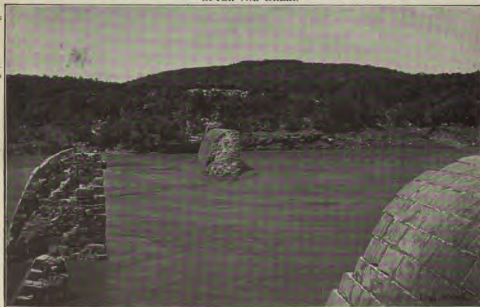
FIG. 231.—AUSTIN DAM, TEXAS, AFTER SUBSIDENCE OF FLOOD OF APRIL 7, 1900. Showing section of masonry moved bodily down-stream.
