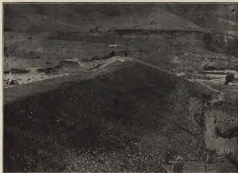
FIG. 133.—DAM No. 1, AT ACATLAN, TENANGO RIVER, COMPLETED JULY, 1906. THE MATERIALS FOR THE DAM WERE GROUND-SLUICED FROM THE BORROW-PITS IN THE BACKGROUND.
