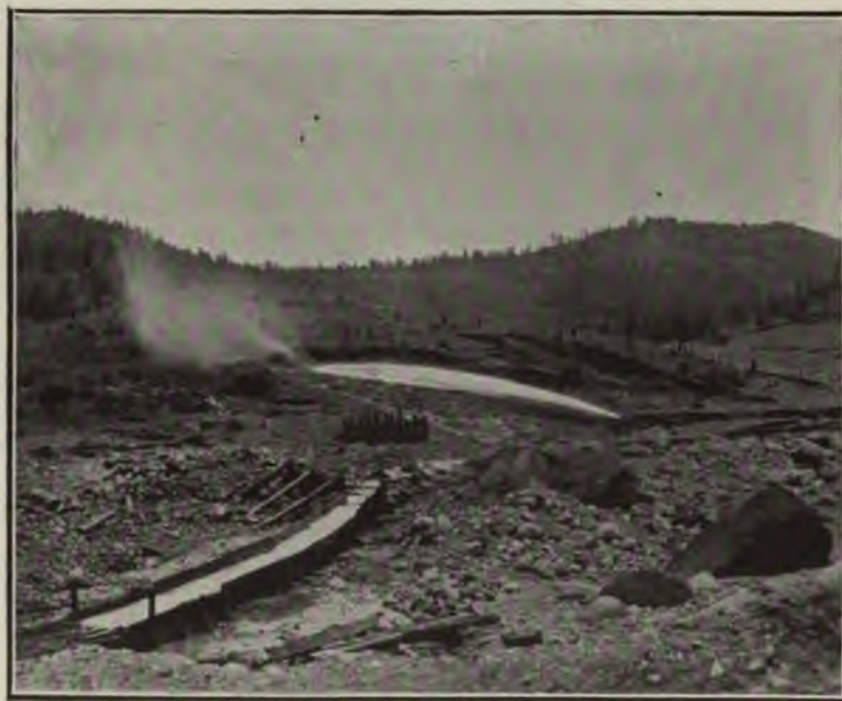
FIG. 103.—HYDRAULIC SLUICING ON THE TERRACE DAM, COLORADO.
