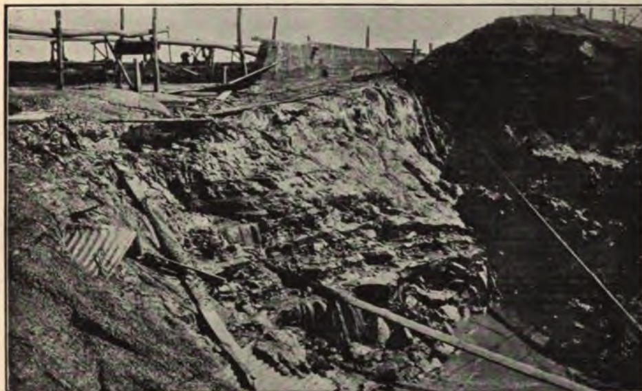
FIG. 377.—ILLUSTRATING THE COMPACT CHARACTER OF THE CLAY CORE OF THE SANTO AMARO DAM, ACCIDENTALLY EXPOSED TO VIEW BY A BREAK FROM THE POND ON TOP OF THE DAM.
