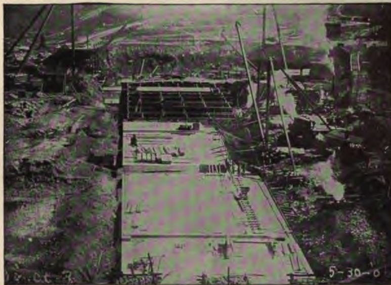
FIG. 320.—FLOOR CONSTRUCTION, JUNIATA DAM.
