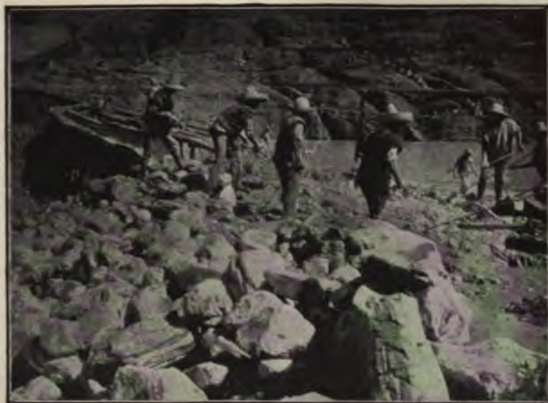
FIG. 118.—STONE CARRIED THROUGH FLUME TO UP-STREAM SLOPE OF THE NECAXA DAM.
