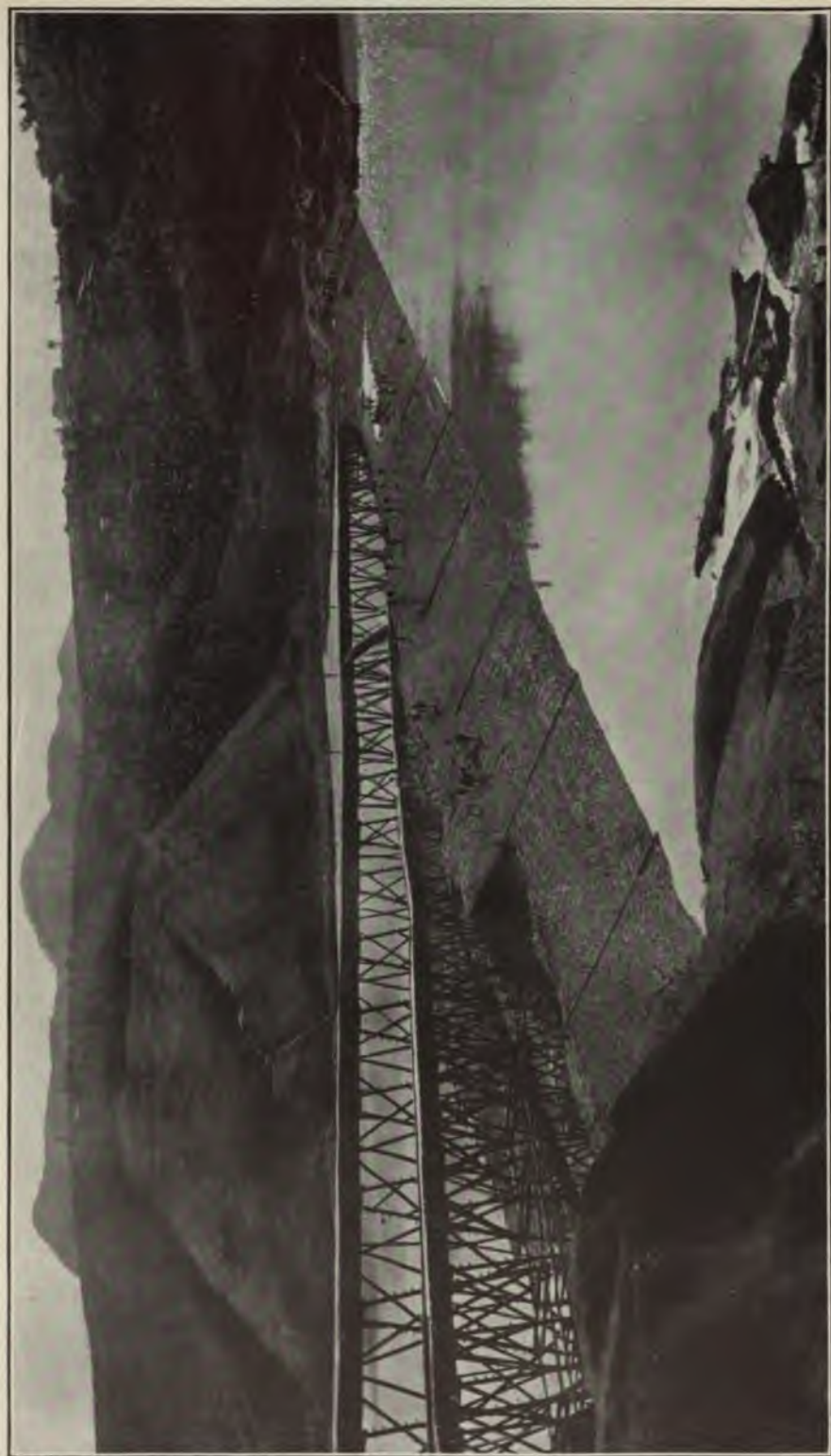
FIG. 129.—UP-STREAM TOE OF NECAXA HYDRAULIC-FILL DAM, DEC. 9, 1907, SHOWING DELIVERY OF MATERIALS BY FLUMES. THE CORE-WALL IS SHOWN IN CENTER OF DAM.
