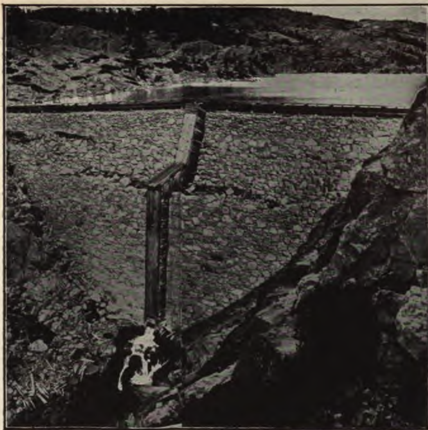
FIG. 343.—THE EUREKA LAKE ROCK-FILL DAM, CALIFORNIA, SHOWING COVERED MAN- WAY TO REACH GATES FROM CREST IN WINTER.
