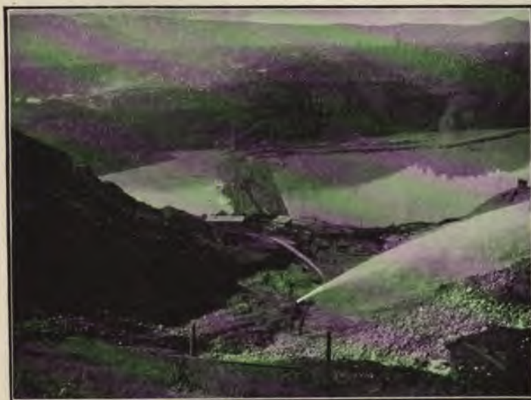
FIG. 116.—HYDRAULIC MONITOR IN ACTION, WITH 30 SECOND-FEET UNDER 180 POUNDS PRESSURE, 6-INCH NOZZLE. UP-STREAM TOE OF DAM SHOWN, WITH TAILING POND AT LEFT.
