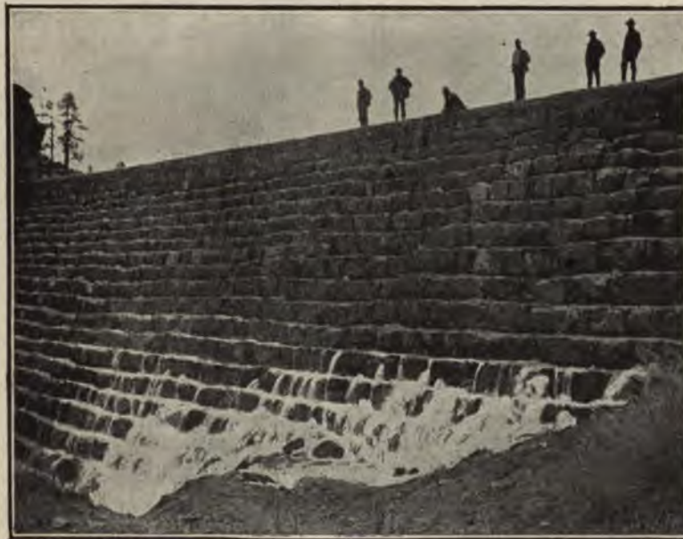
FIG. 30.—CASTLEWOOD DAM, COLO., SHOWING LEAKAGE THROUGH ROCK-FILL.
