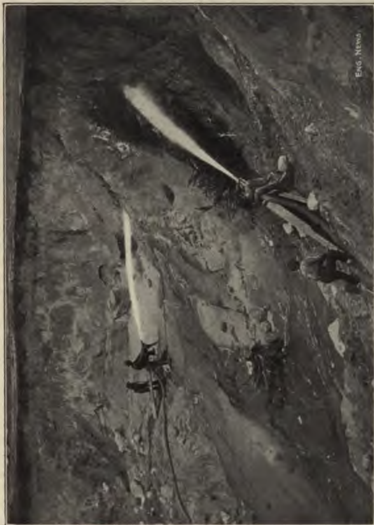
FIG. 139.—HYDRAULIC SLUICING ON THE CROTON DAM, SHOWING THE IMPROVISED NOZZLE CONTROL, OR HYDRAULIC MONITOR.
