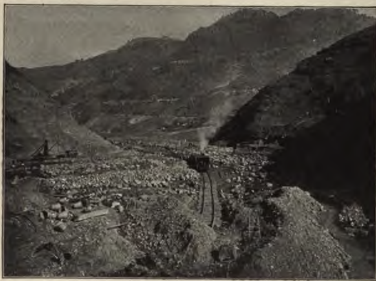
FIG. 114.—LOOKING UP STREAM AT SITE OF DAM NO. 2, AT NECAXA, SHOWING STRIPPED ABUTMENTS FOR THE DAM ON EACH SIDE.
