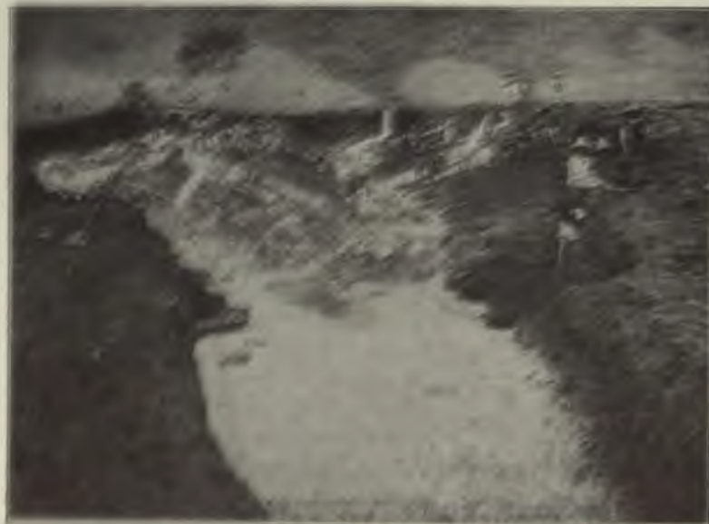
FIG. 131.—GROUND-SLICING ON DAM NO. 1, TENANGO RIVER.
