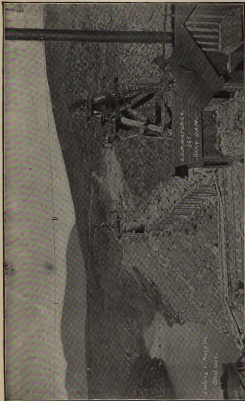
FIG. 13.—OTAY (CAL.) ROCK-FILL DAM—STEEL CORE.
