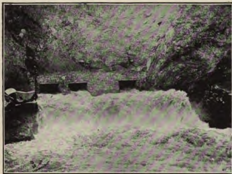
FIG. 97.—WAIĀLAE DAM, HAWAII, SHOWING FLOOD DISCHARGE THROUGH OUTLET TUNNELS DURING CONSTRUCTION, UNDER HEAD OF 8 FEET AT UPPER END OF TUNNELS.
