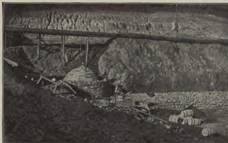
FIG. 87.—DOME ON GATE CHAMBER, LAKE FRANCES DAM; ALSO TWENTY-TWO-INCH SLUICE PIPE.
