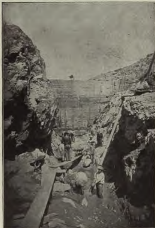
FIG. 11 —MASONRY FOUNDATION OF LOWER OTAY DAM.
