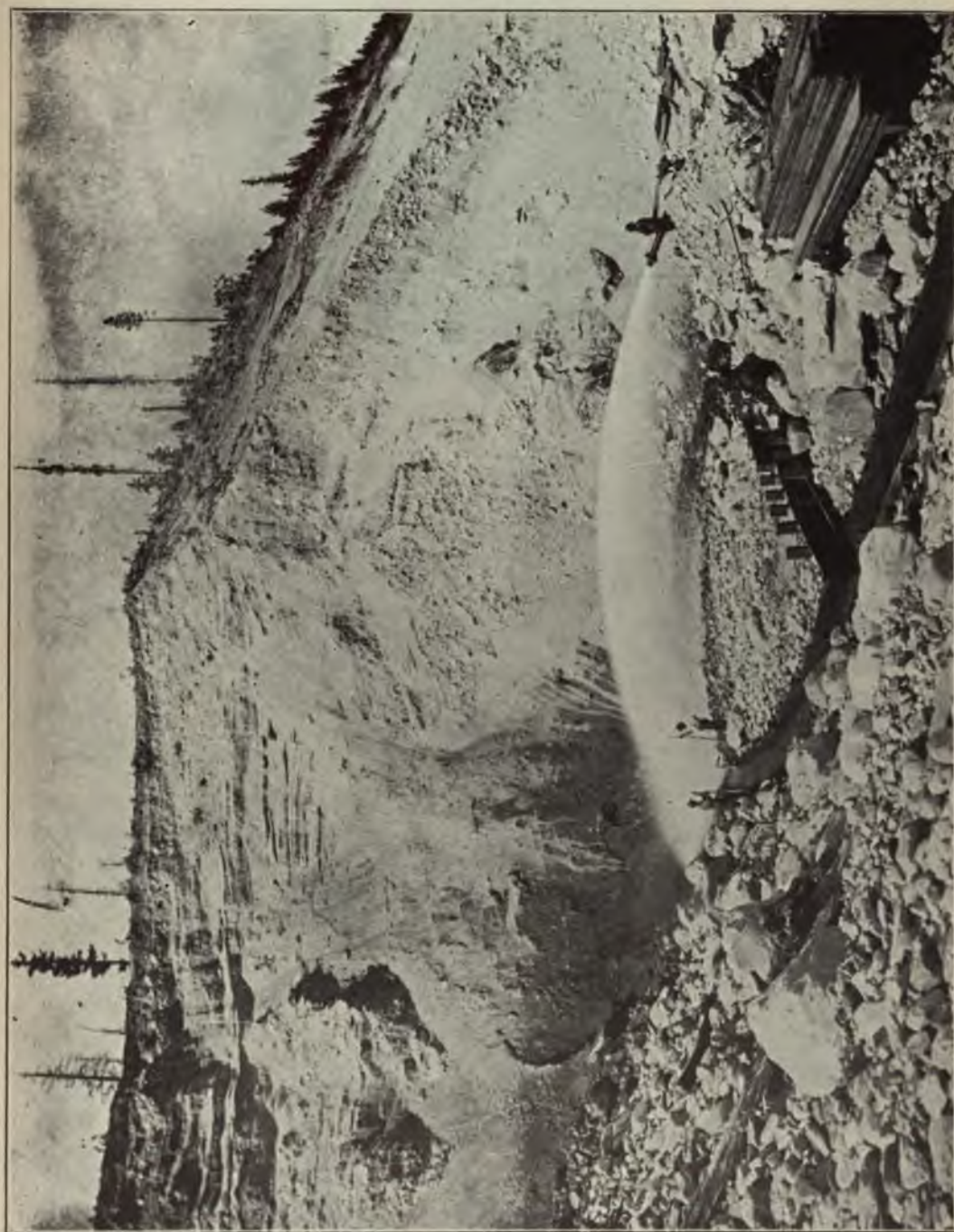
FIG. 140.—HYDRAULIC SLUICING, CANADIAN PACIFIC RAILWAY. VIEW OF PIT, AND HYDRAULIC GIANT AT WORK.
