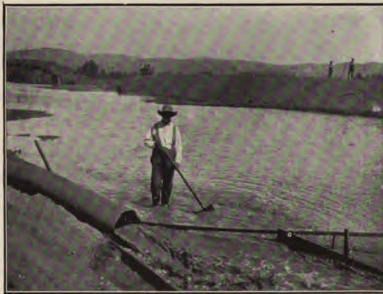
FIG. 135.—YORBA DAM, CALIFORNIA. SHOWING DISCHARGE OF PUMPED MATERIAL, ALONG UP-STREAM TOE LEVEE.
