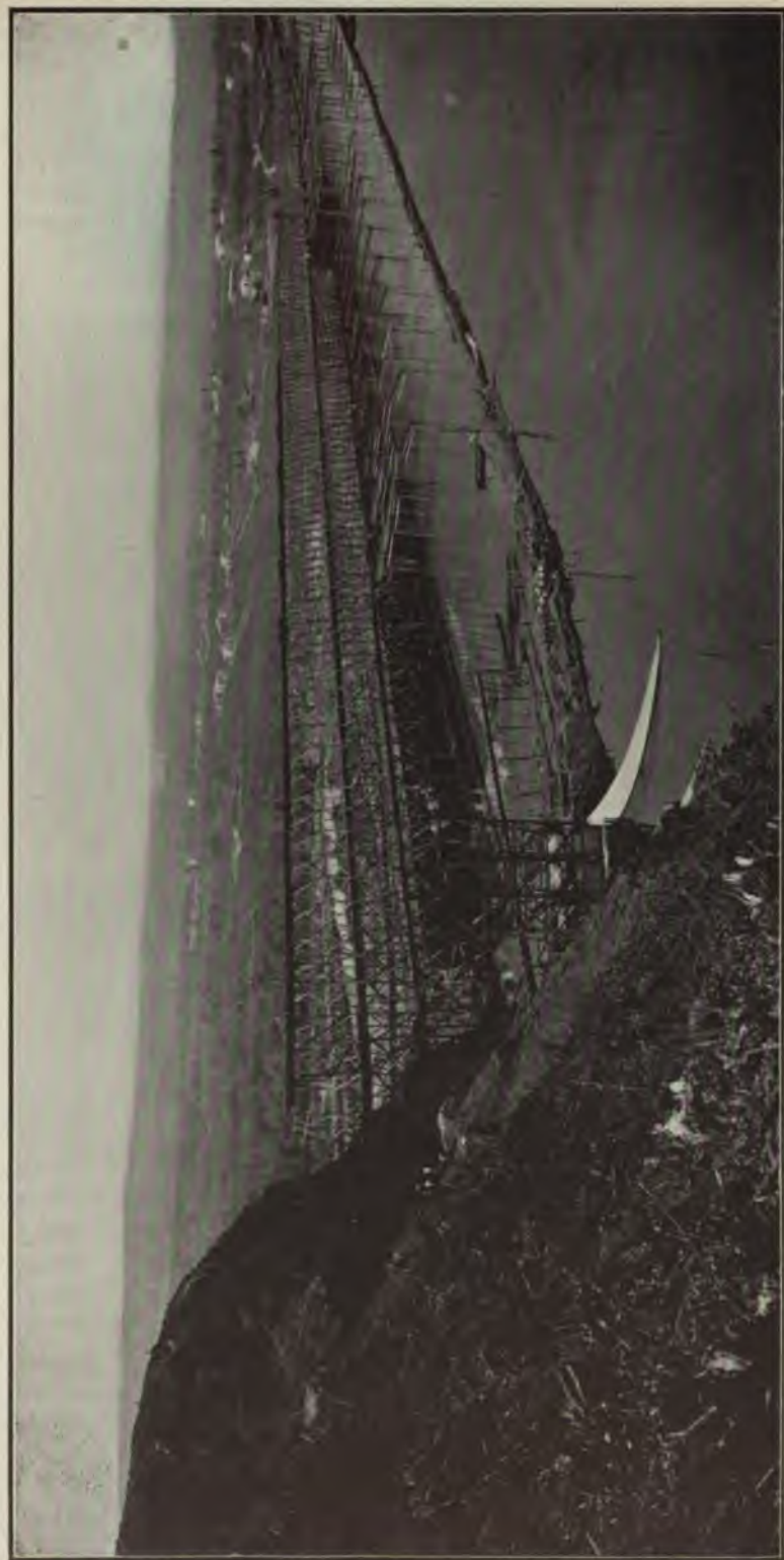
FIG. 109.—GENERAL VIEW OF SANTO AMARO DAM, BRAZIL, AUG. 21, 1907. SHOWING THREE LEVELS OF DELIVERY ON CENTRAL TRESTLE. TOTAL LENGTH 5300 FEET, MAXIMUM HEIGHT 63 FEET. TOTAL 148
