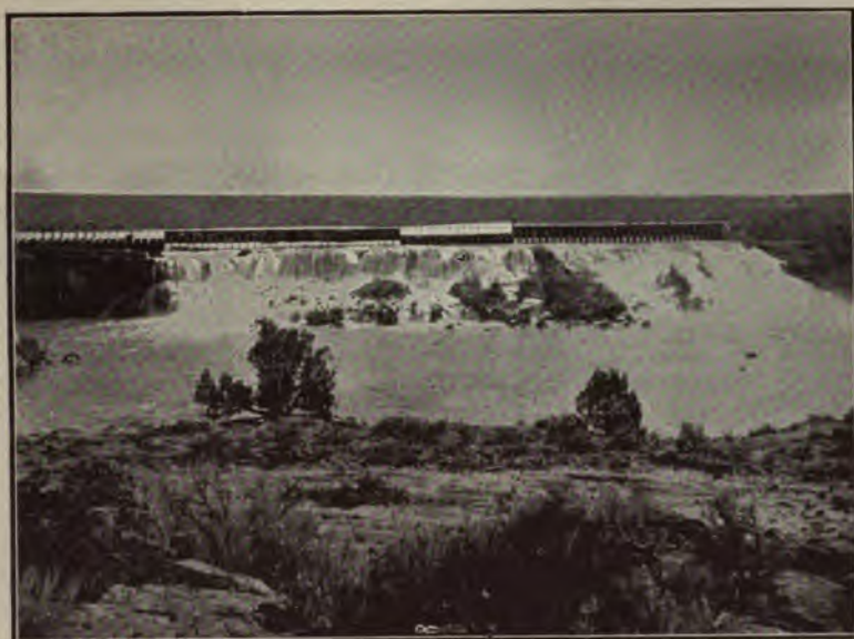
FIG. 47.—MILNER DAM, SNAKE RIVER, IDAHO. DISCHARGE THROUGH THE GREAT BATTERY OF 99 WASTE-GATES FORMING "IRRIGATION FALLS," 40 FEET HIGH.
